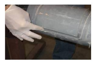
The wearpad is pushed into position on the pipe. Any excess FibaGel can be then be wiped away. This will leave a FibaGel seal along the edge of the wearpad. Both 120° and 90° WearPads will require strapping whilst the adhesive cures to hold the wearpad in place. Ensuring that the wearpad is tight and secure against the pipe, the pipe can then be lowered into place.
