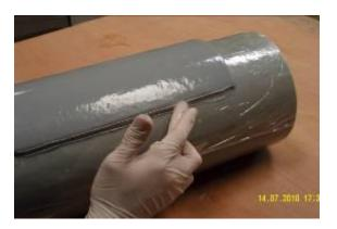
The bead can then be smoothed using a damp gloved finger to create a good edge seal.
