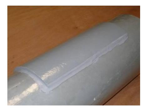
Both 120° and 90° WearPads will require strapping whilst the adhesive cures to hold the wearpad in place. Ensuring that the wearpad is tight and secure against the pipe, the pipe can then be lowered into place.
