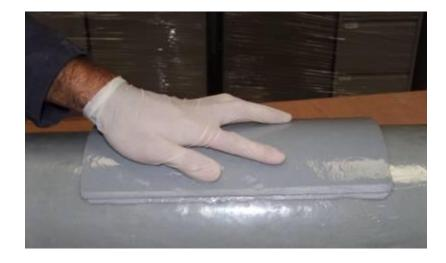
A bead of FibaBond should be applied to the outer edge of the pad to ensure a full waterproof seal to the pipe.
